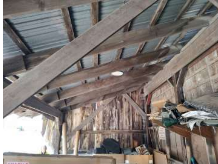
Final View of inside existing 3-Bay Work Zone
