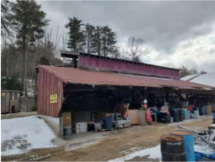
Front View of 3-Bay Work Zone Area
