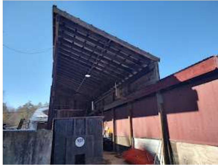
Back Wall of Work Zone Area
