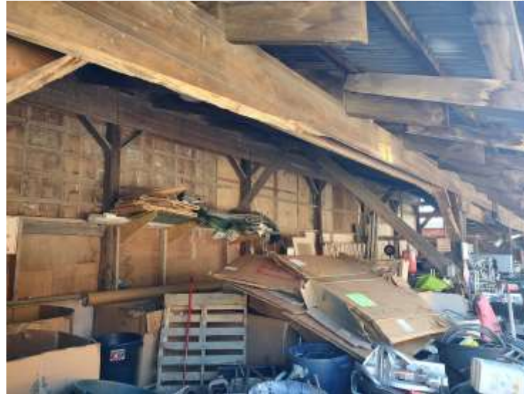
Inside existing 3-Bay Work Zone
