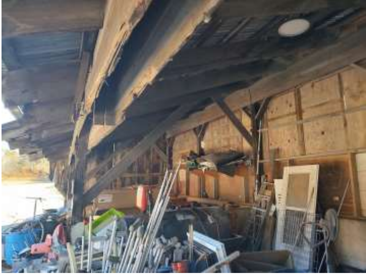
Inside existing 3-Bay Work Zone
